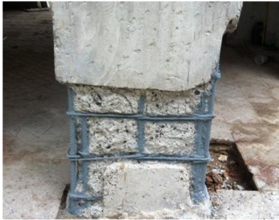
TYPICAL IMAGE OF SURFACE PREPARED RCC MEMBER
